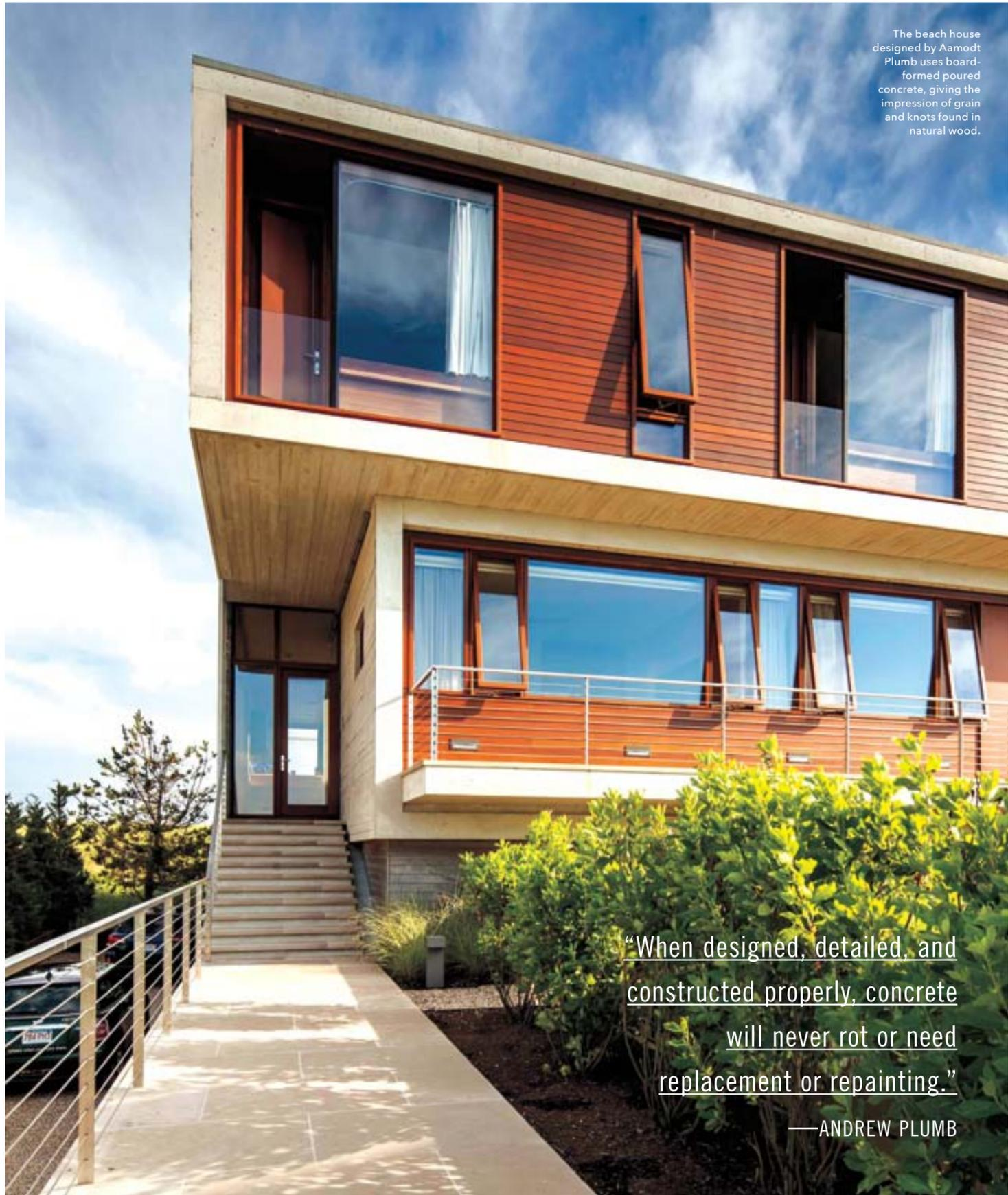
The beach house designed by Aamodt Plumb uses board-formed poured concrete, giving the impression of grain and knots found in natural wood.
